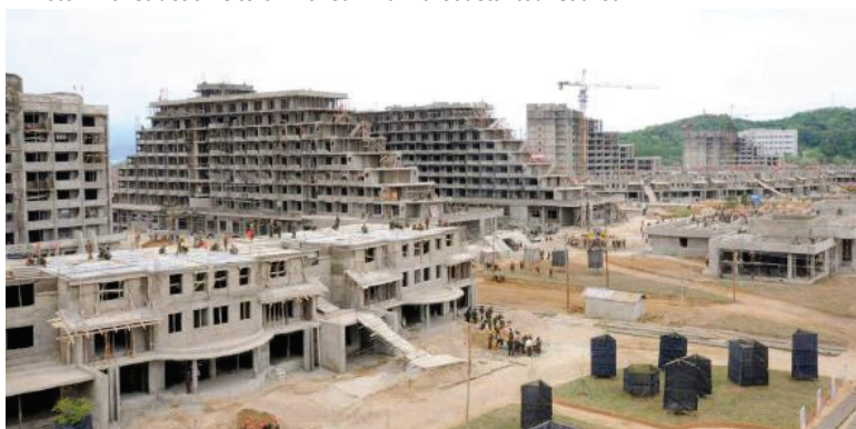
<Photo> Construction site of Wonsan-Kalma coastal tourist area
